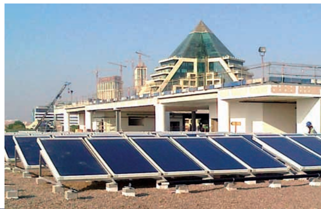
AL-JALILA HOSPITAL - Dubai (EAU) 50 pannelli - 135 mq Acqua calda sanitaria
